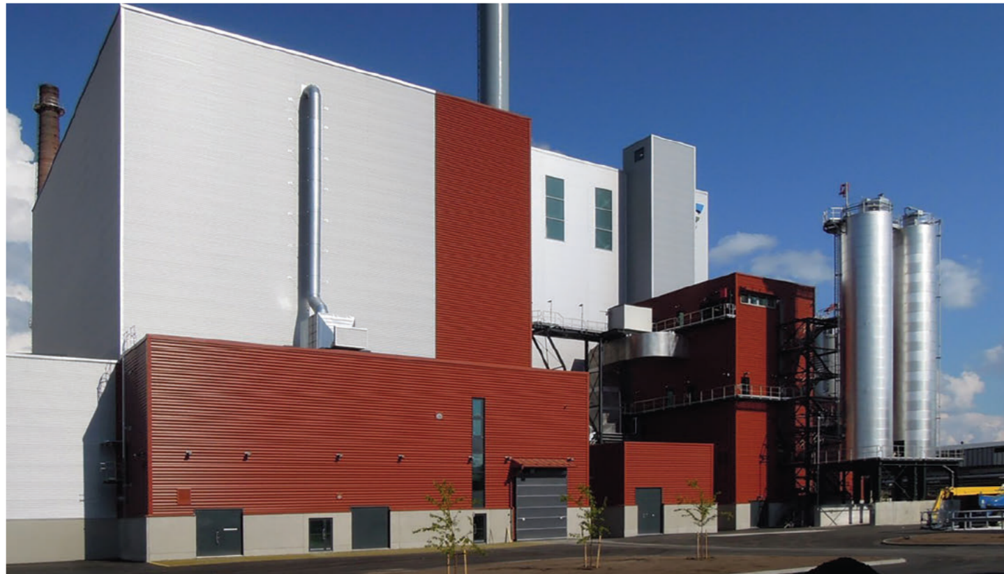
Example EfW facility already constructed using the proposed EfW technology provider
